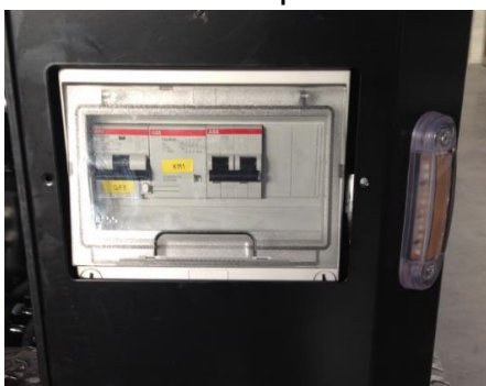
15. Main differential panel
