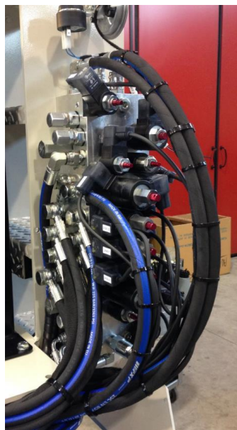
14. Main hydraulic unit
