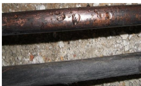
Damaged hydraulic hose pipe
