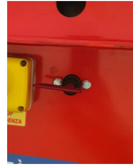
14. Battery disconnect switch
