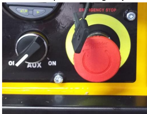
9. Ground control panel emergency button
