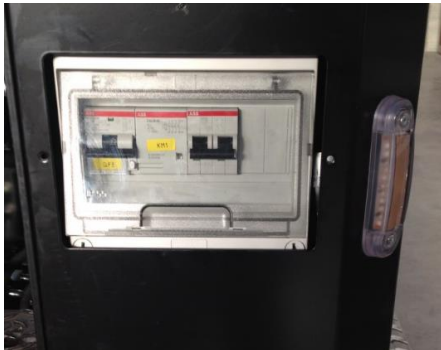
15. Main differential panel
