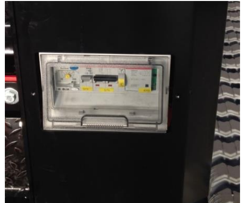
32. Inverter differential panel (if present)
