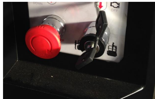
21. Ground control panel emergency button
