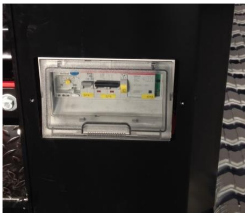
34. Inverter differential panel (if present)
