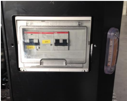
18. Main differential panel
