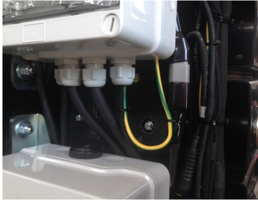
22. ECU electronic control unit
