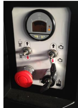
19. Ground control panel
