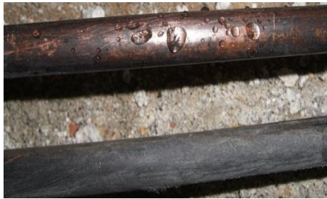
Damaged hydraulic hose pipe
