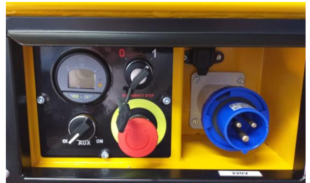
6. Ground control panel
