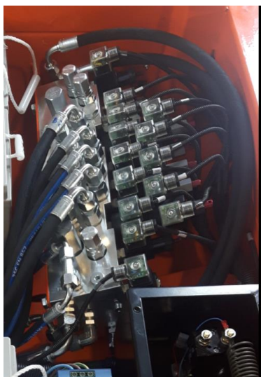
7. Main hydraulic unit
