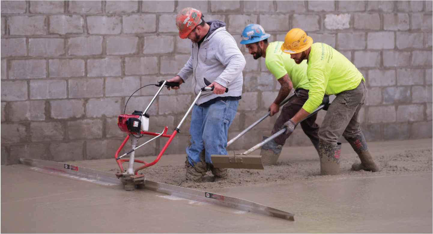
The unique, patented blade simultaneously cuts and smooths concrete.
