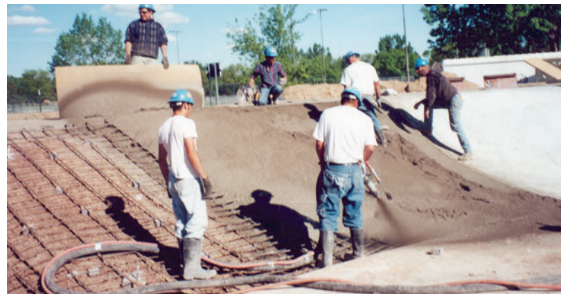
Shotcreting (wet gunning) with a stiff, low-slump shotcrete mix is all in a day's work for the Mayco C30HD.
